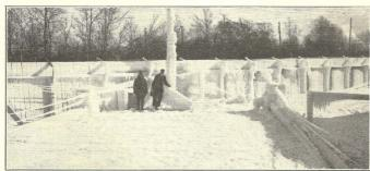
A VIEW IN FRONT OF THE PROPELLER RIG, AFTER A SIX-HOUR WATER-SPRAY TEST
